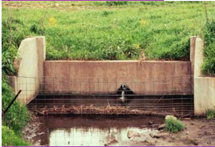
Figure 7.14 Grade Stabilization Structure (USDA-NRCS)
